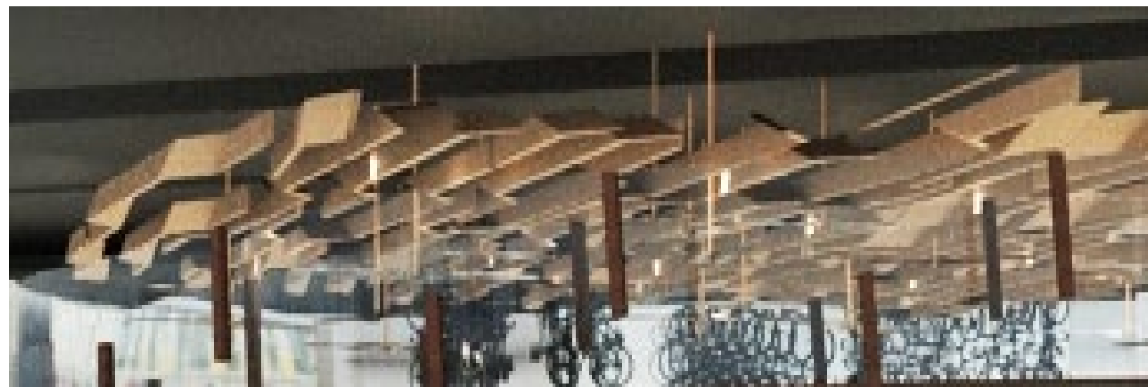
Install 3D shapes on the ceiling, cooperate with fans to increase air flow
